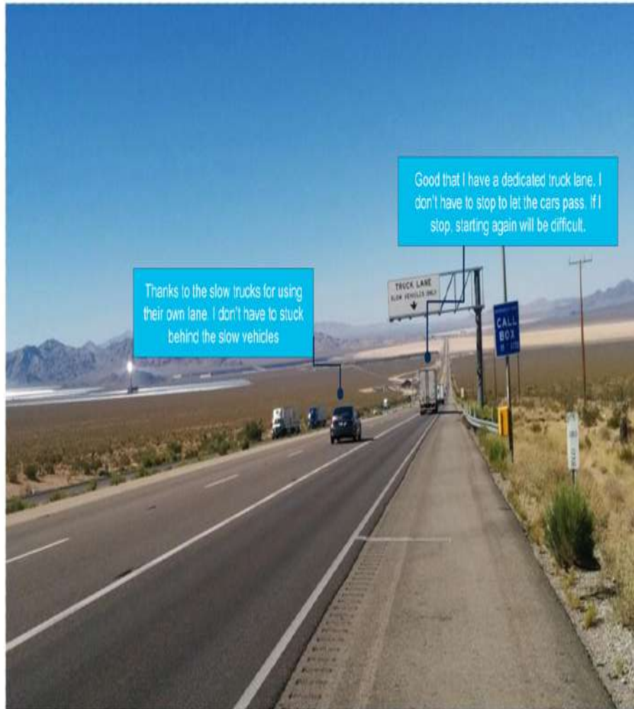
Figure 6-5 Traffic and congestion segregation to dedicated lanes.
